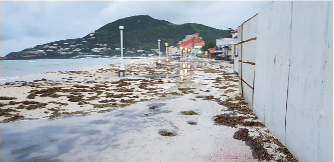
Impact of Surge on Boardwalk in Philipsburg: September 24 th 2019
